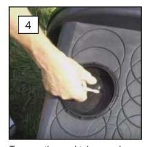
To open the seal tabs us a key or screwdriver to start the pull tab for the correct pipe size.
